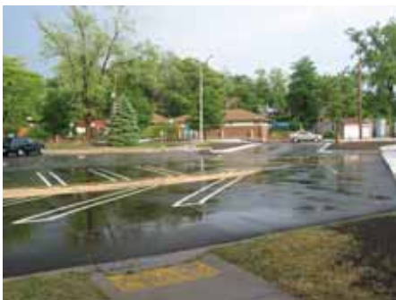
Infiltration BMPs installed at Washington Park
